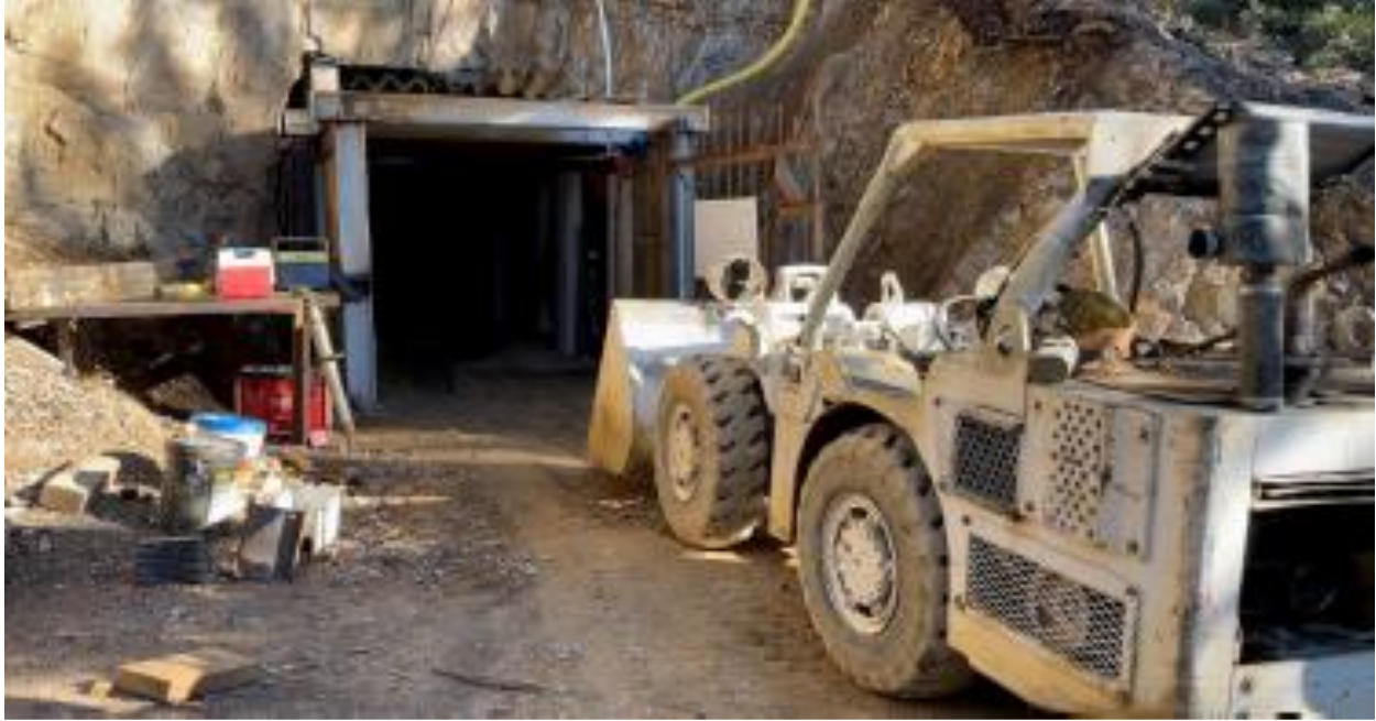
Picture 1. Mt. Vernon Main Portal
