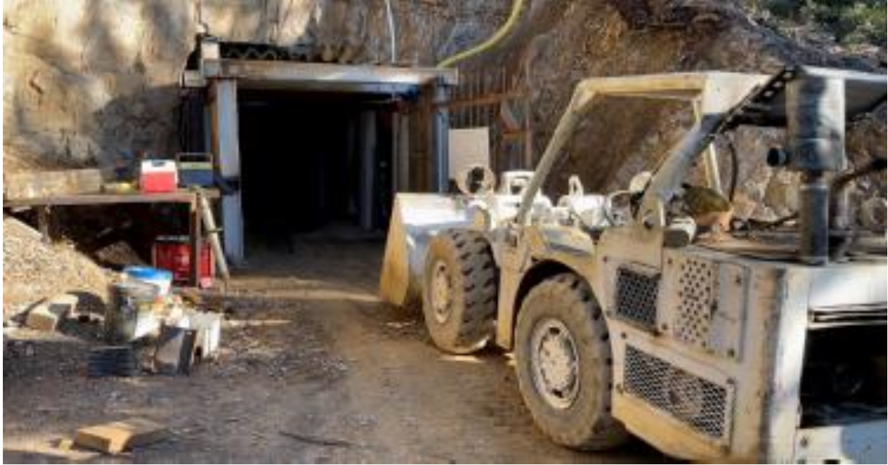
Picture 1. Mt. Vernon Main Portal
